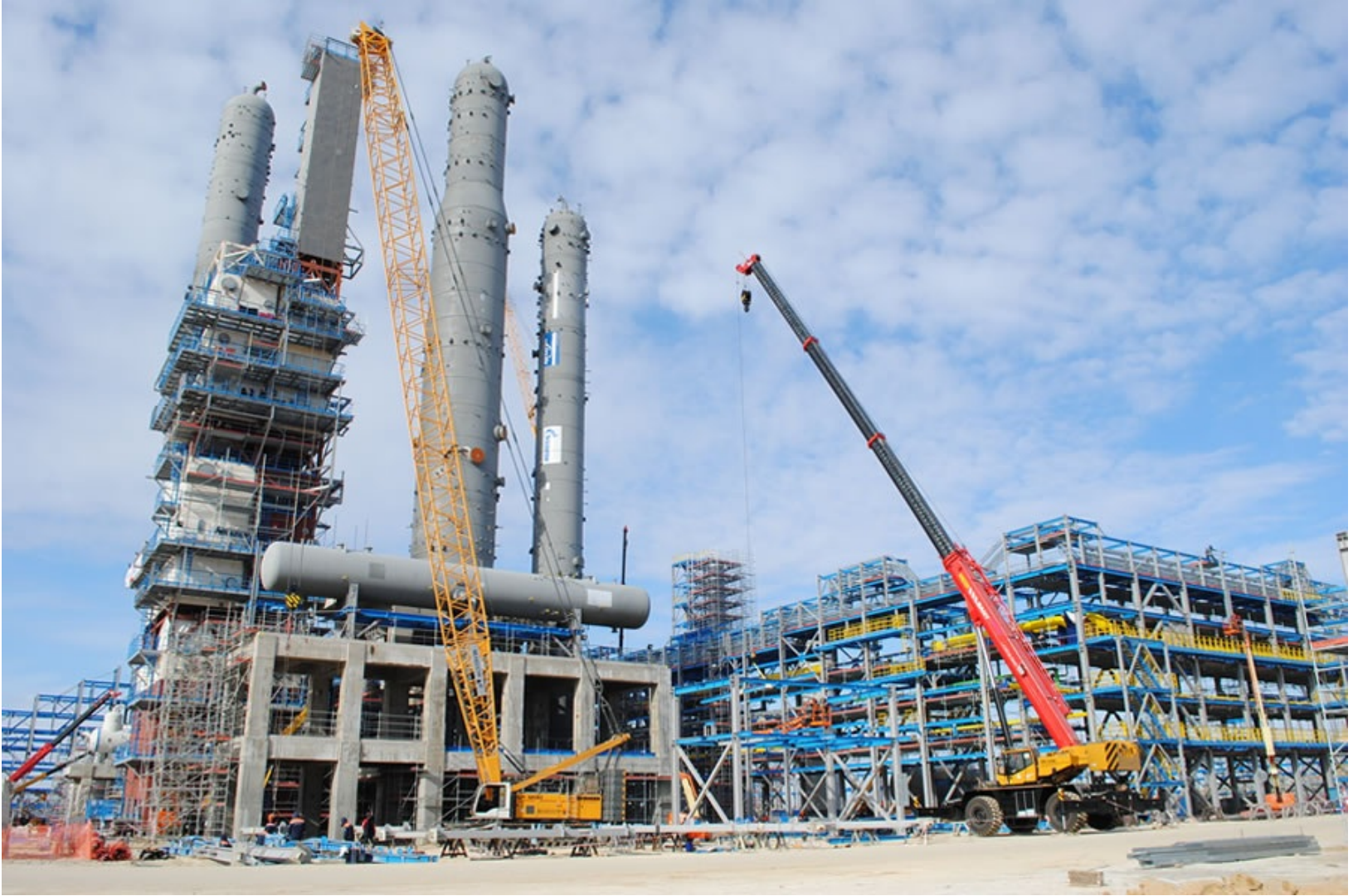
Amur GCC construction.
